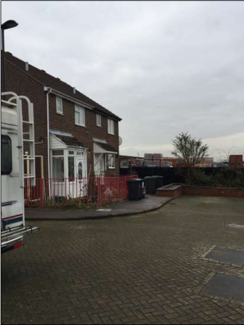
Views from The Green (rear of site)
